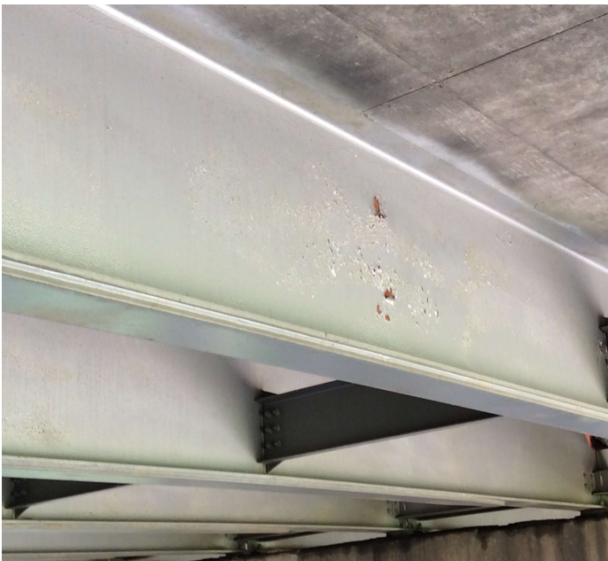
PHOTO 1 Description Paint. Span 1. Beam 5.
