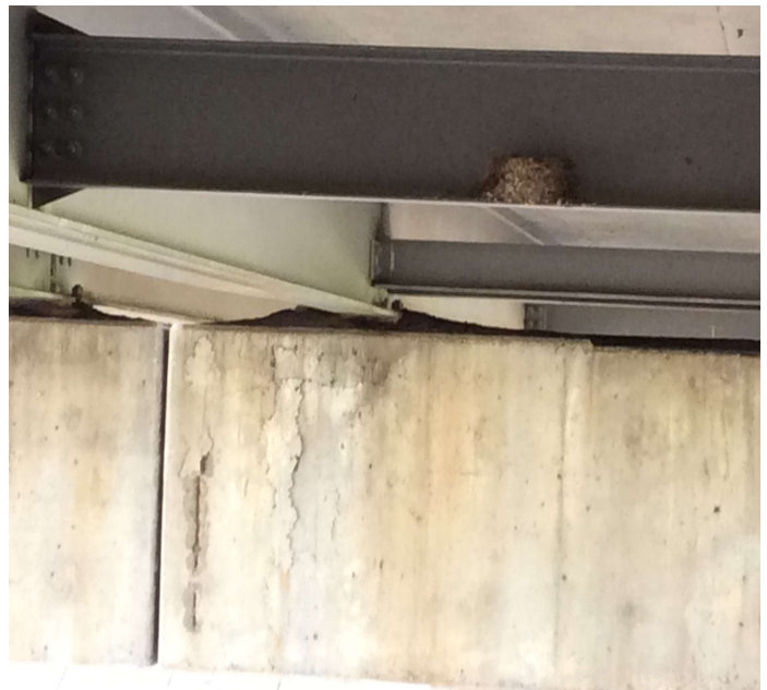
PHOTO 2 Description Debris on bent 2 cap.
